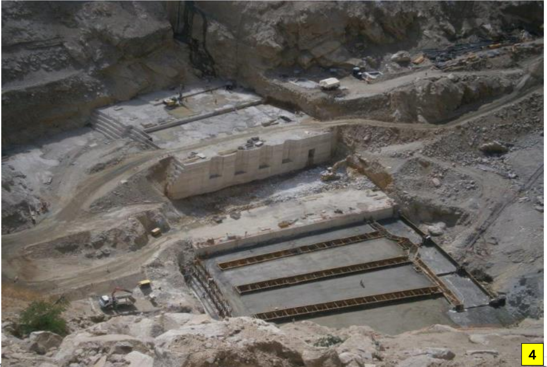
Dam Excavation (Right Margin)
